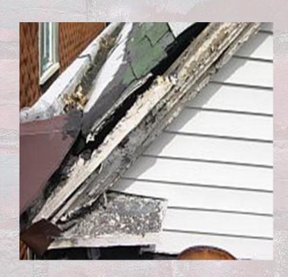
Wood Rot. Common in windows, soffits, eaves, and on siding.
